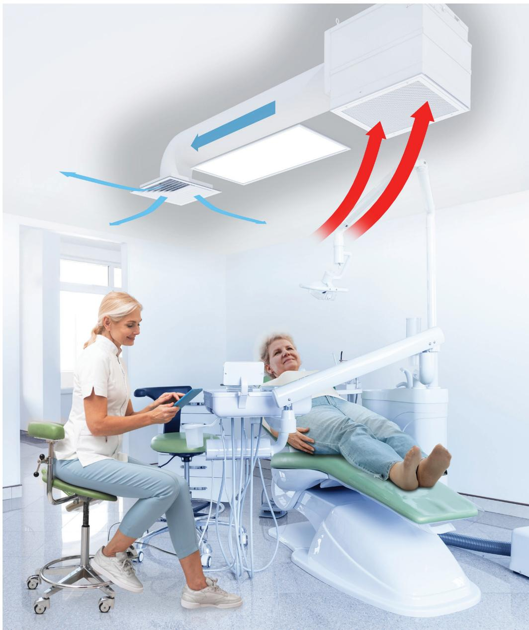
contaminated air is drawn away from the dental practitioner, and filtered air should be supplied from behind the patients head to wash the work space with clean air.
