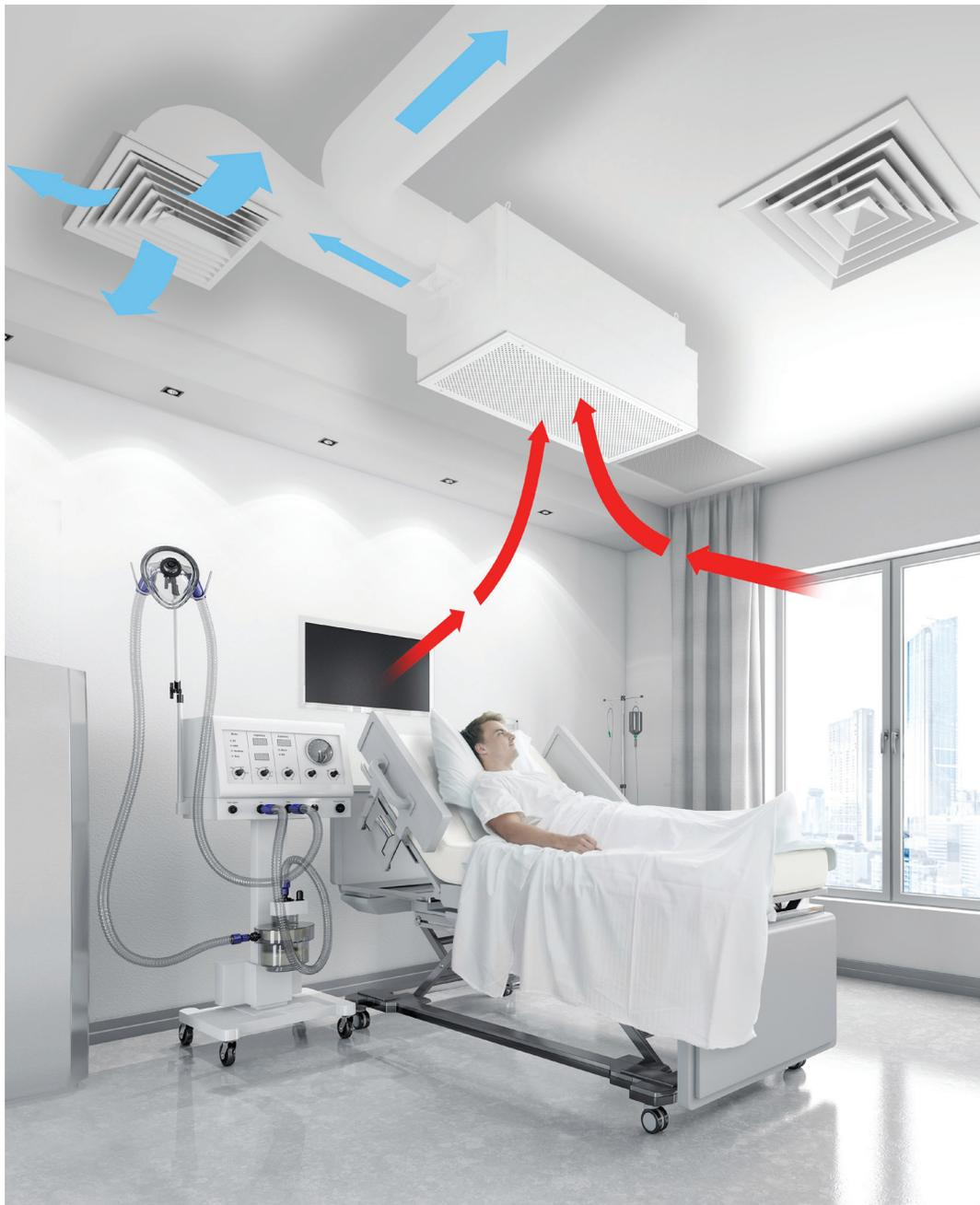
In these applications the Puraflo should be located directly over the patients head so that contaminated air is drawn directly out of the room, and filtered air should be supplied toward the door so that airflow is encouraged to move from clean to less-clean areas of the room.
